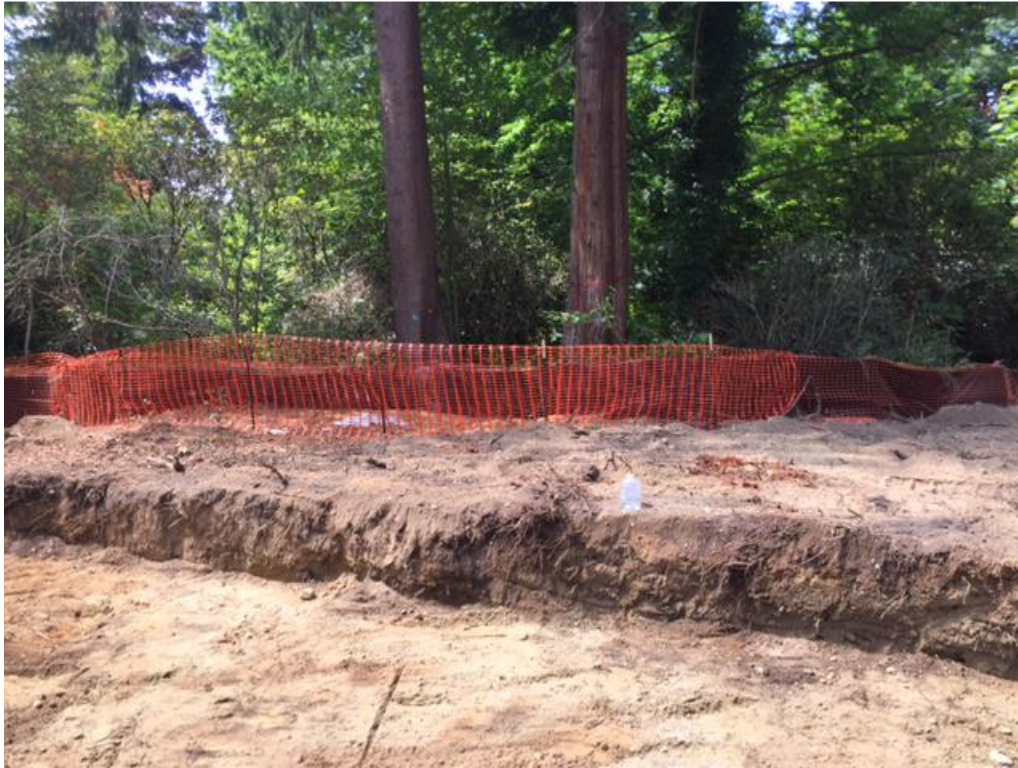
Image from 2018 showing trench east of trees #8409 and #8410
