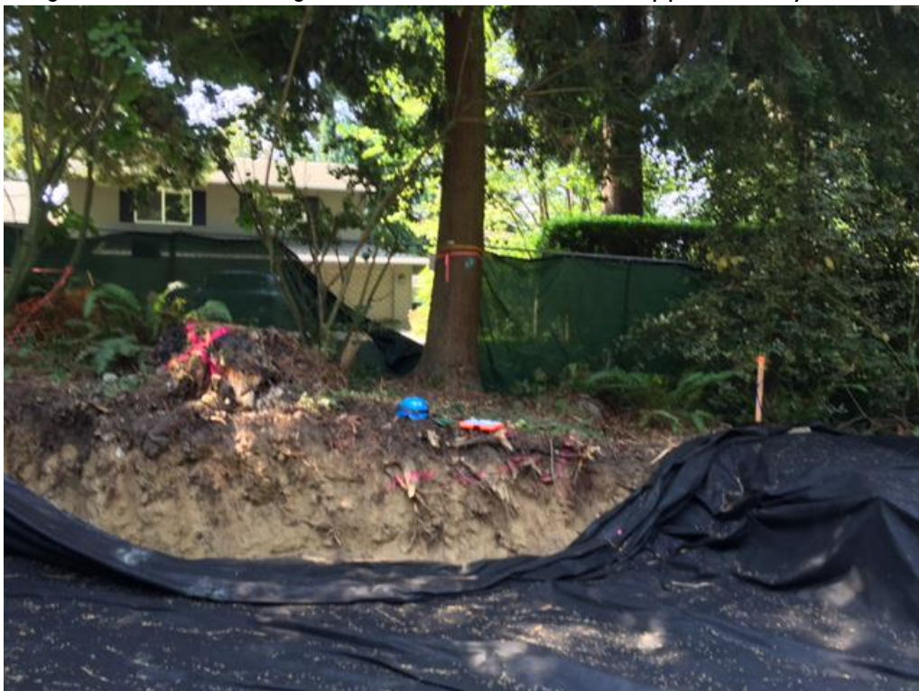
Image from 2018 showing Tree #8251 with roots torn approximately 8' north of the trunk.
